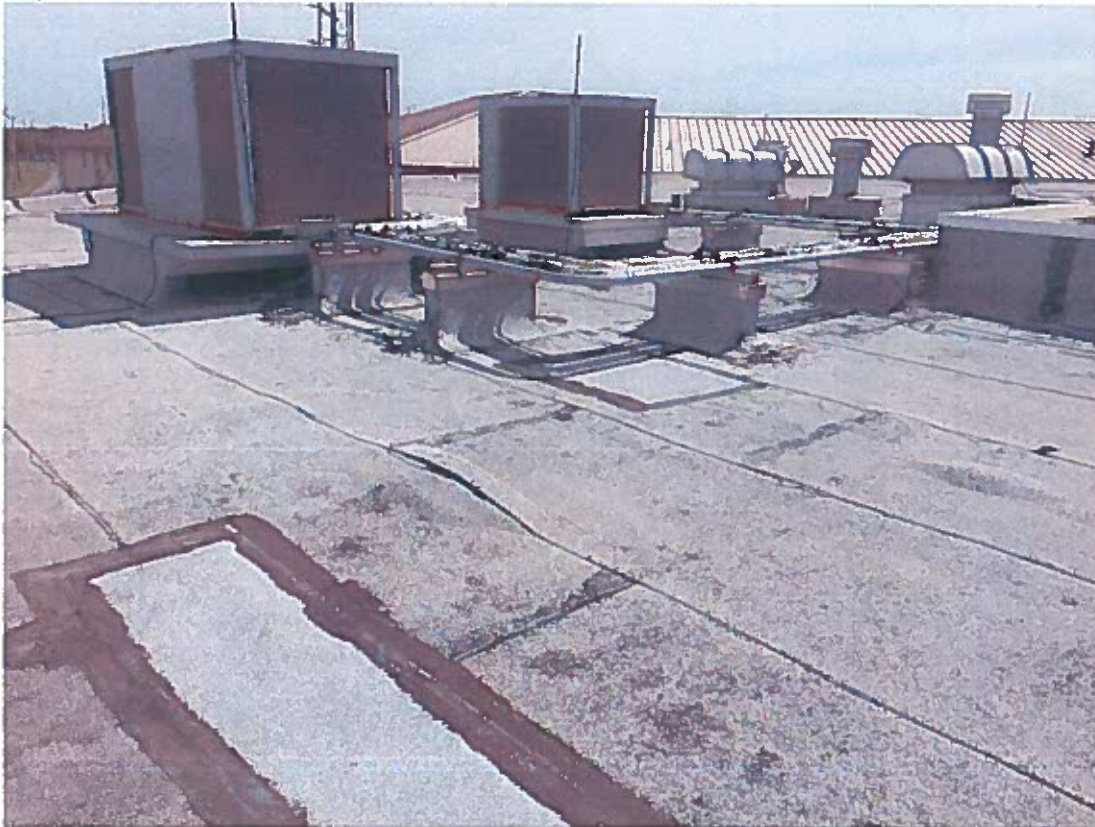
One of two of existing split DX units to be resized and replaced with smaller DX units.
