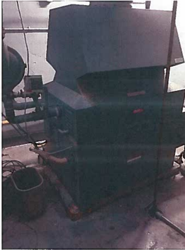
SPACE HEATING: Provide heat pump DX units and demolish hydronic space heating system.
