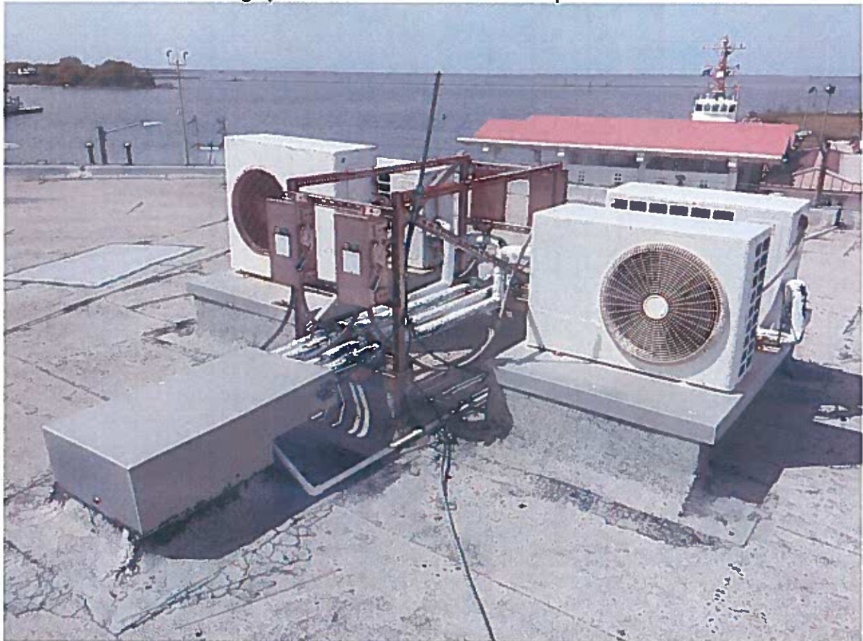
Four DX units serving 2 nd floor to be demolished. Six new DX units (split and package) to be provided for space cooling and heating.
