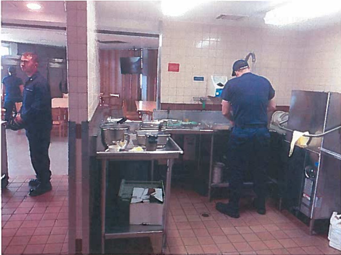
HOBART dishwasher without hood to be replaced in one day with ventless warewasher with cold water.
