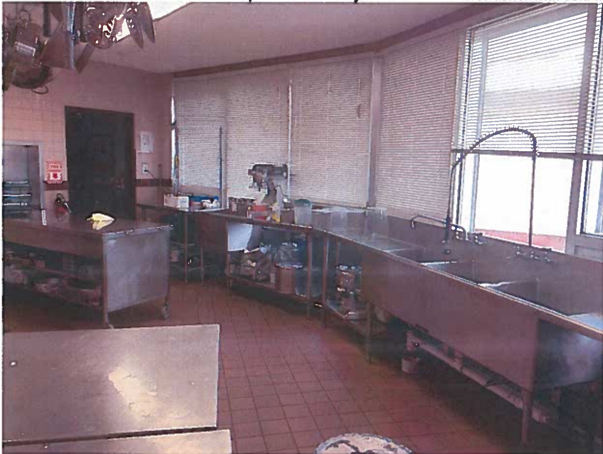
Wash sink requires new drain line and grease trap.
