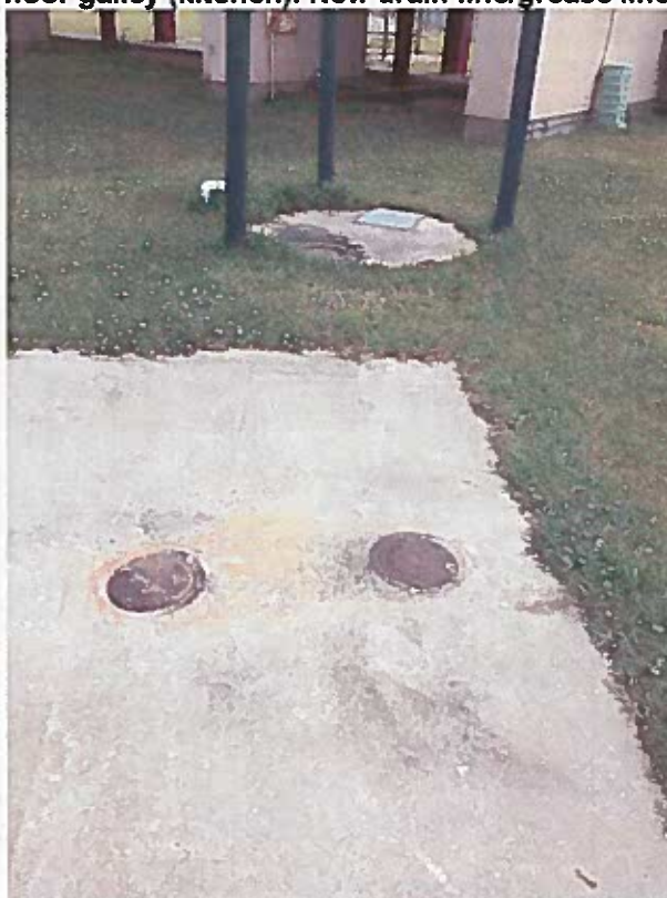
New drain line/grease line from sink to under-ground grease interceptor required.
