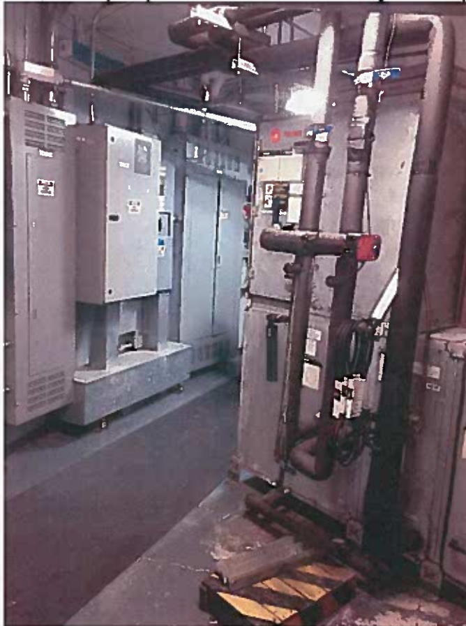
One of two of existing split DX units to be resized and replaced with smaller DX units.
